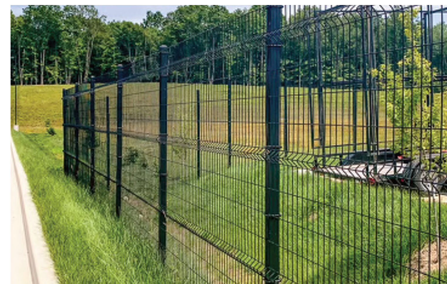
PANEL FENCE - REPAIR EXISTING AND ADD ADDITIONAL GATES ALONG WEST ENTRANCE
